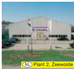
NL Plant 2, Zeewolde
